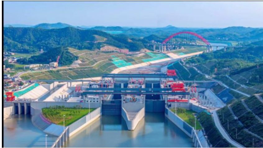
Figure 2. Drone photo of the Ma'dao navigation hub of the Pinglu Canal, Guangxi 2
