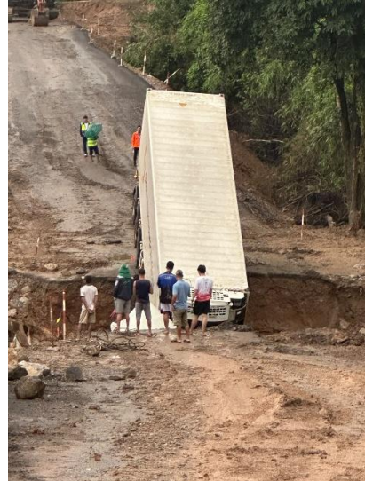
Figure 3. Damage to the Houay Pasouan bridge near Ban Done in late June 2026 and flood damage to the bypass culvert in early July 2026 (Photos courtesy SilviCarbon). Although a temporary dirt diversion culvert was built, heavy rains washed it away by early July. Long-term reliance on a dirt bypass during the monsoon season has proven unviable, stranding hundreds of bonded trucks on both sides of the crossing and paralysing transit between Central Laos and Vietnam. A new concrete bridge is currently under construction and is expected to be completed about February 2027.
