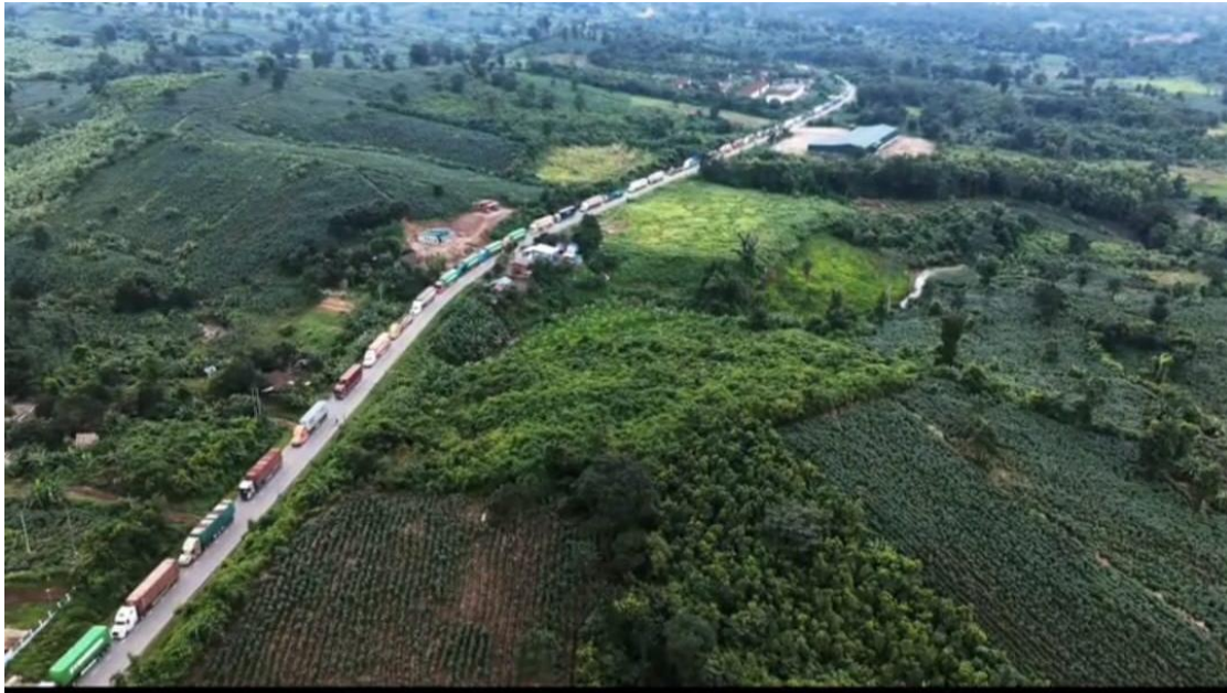
Figure 5. Huaypaxuan bridge on National Road No. 9 Temporary causeway flooded. Causing long and serious queues and delays. 13 September 2026.
