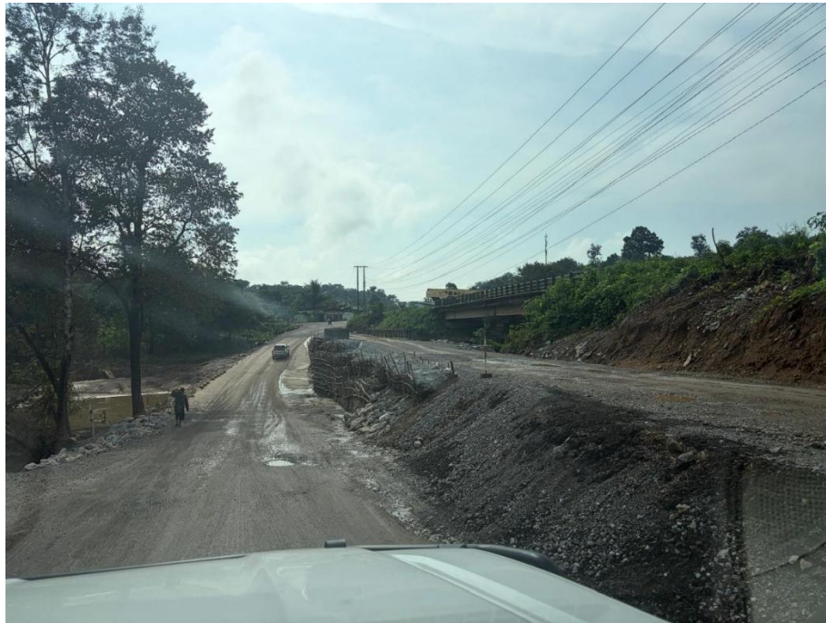
Figure 4. Temporary bridge diversion 17 September 2026.
