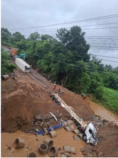
Figure 3. Damage to the Houay Pasouan bridge near Ban Done in late June 2026 and flood damage to the bypass culvert in early July 2026 (Photos courtesy SilviCarbon). Although a temporary dirt diversion culvert was built, heavy rains washed it away by early July. Long-term reliance on a dirt bypass during the monsoon season has proven unviable, stranding hundreds of bonded trucks on both sides of the crossing and paralysing transit between Central Laos and Vietnam. A new concrete bridge is currently under construction and is expected to be completed about February 2027.
